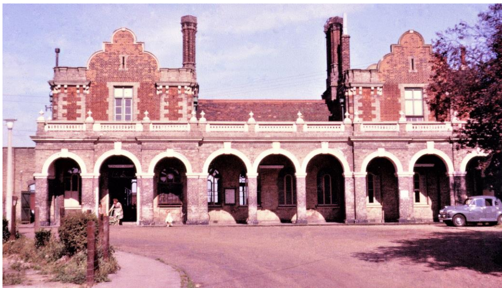
Maldon and Heybridge Station exterior
