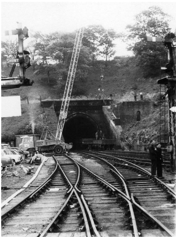
The crane in action probably on a Sunday morning
